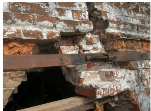
**Fig. 10. Steel bandage around the base of the vault over the second tier**
