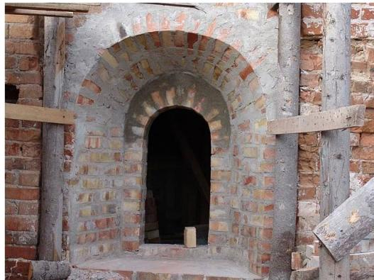
**Fig. 13. Restoration of window lintels**
