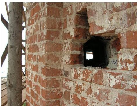
**Fig. 7. Void inside the wall from rotten wooden bandage around the base of the fallen vault over first tier**
