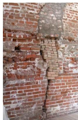
**Fig. 4. Typical vertical cracks – voids stuffed with temporary brickwork**
