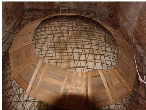
**Fig. 9. Reinforcing cage for concrete vault over first floor**
