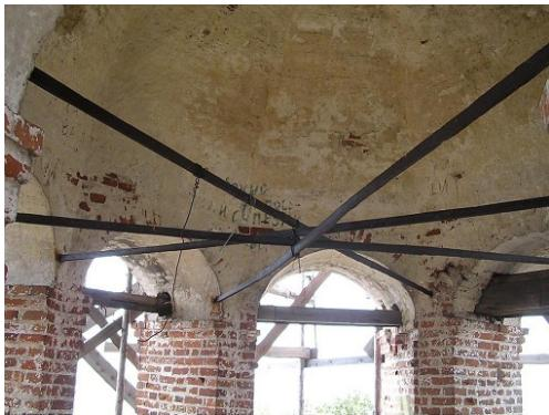
**Fig. 5. Later metal ties, installed in 19 c.**
