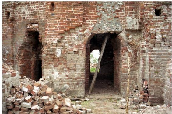
**Fig. 6. Destroyed lintels over doors and windows**
